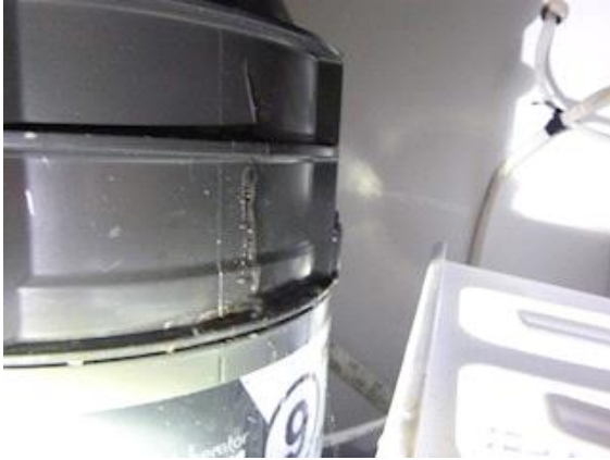
Kitchen: View showing leaking garbage disposal
