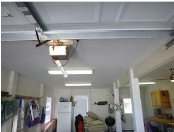
Under Floor Framing & Support: View of garage ceiling panels covering the floor joists
