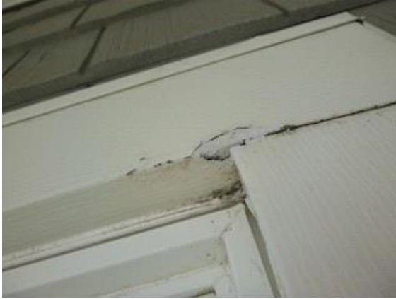
Exterior Surface: View showing corroded trim
