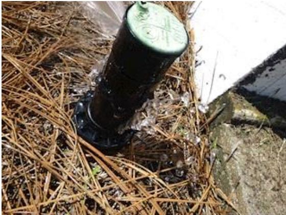
Irrigation System: View showing water leaking from the side of the sprinkler head
