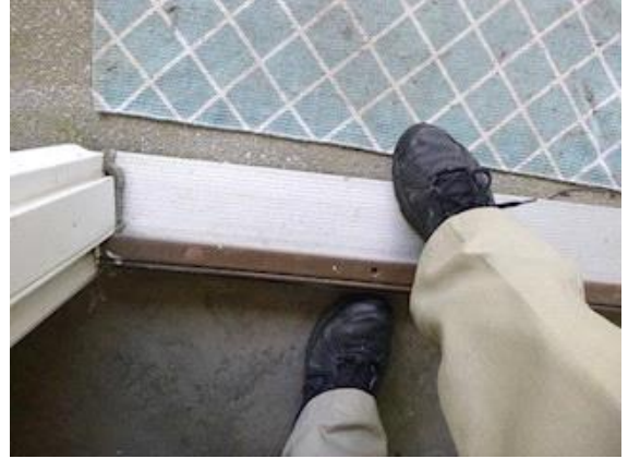
Exterior Doors: View showing loose threshold
