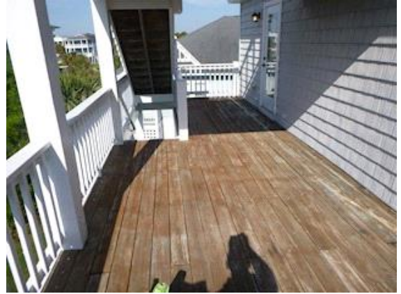
Decks - Rear: Overall view of rear wood deck
