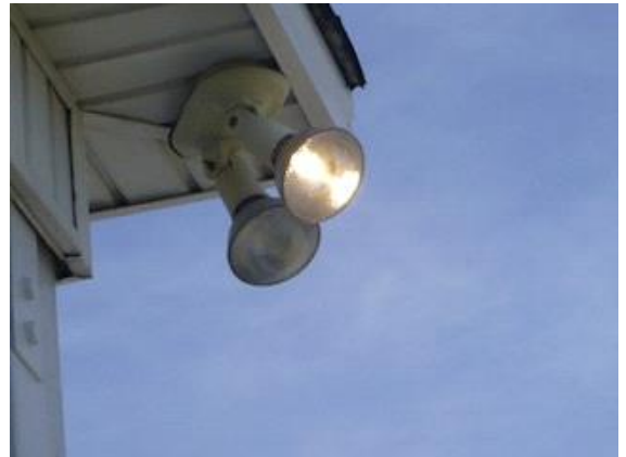
Exterior Surface: Views showing defective exterior lights
