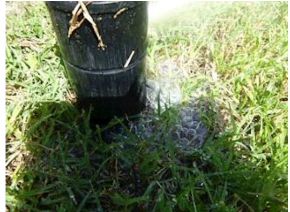
Irrigation System: View of water pooling at the base of the sprinkler head
