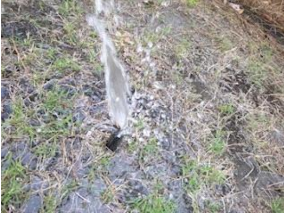
Irrigation System: View showing water spraying from the top of the sprinkler head
