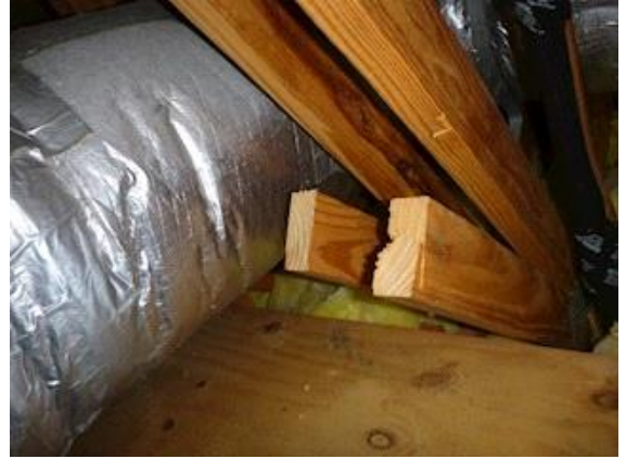
Attic Framing/Sheathing: Views showing cut roof trusses
