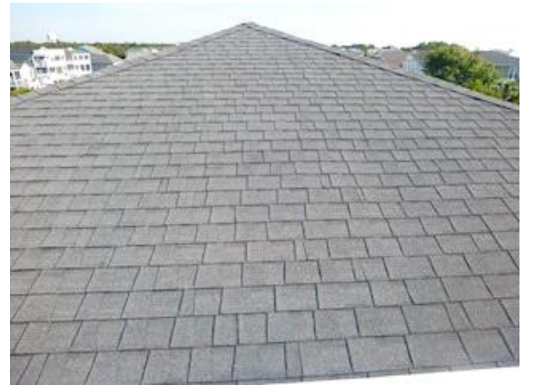
Roofing: Overall views of asphalt roof shingles
