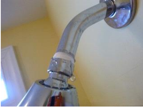
Bathroom #2 - 2nd Floor - Guest: View showing leaking shower head
