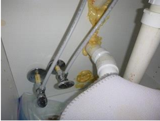
Plumbing: View of plumbing pipes below sinks
