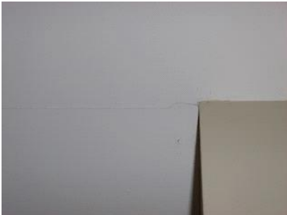
Stairs / Railings: View showing minor drywall crack at the top of the steps
