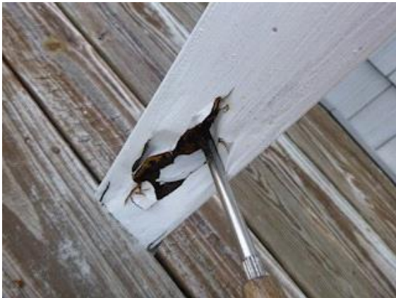
Exterior Doors: View showing water-damaged door core
