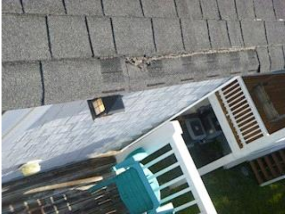
Roofing: Views showing missing shingles
