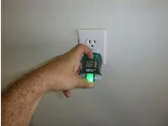
Garage/Under House: View of electrical tester indicating the receptacles are not GFCI protected
