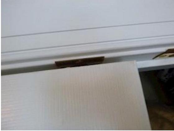
Bedroom #4 - 2nd Floor - Rear/Right: View showing closet door not latching when closed
