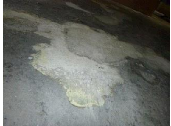
Garage/Under House: View showing efflorescence on garage concrete floor
