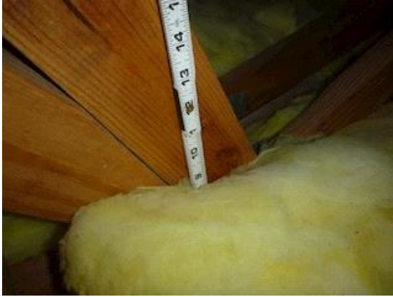
Attic Insulation: View showing the depth of insulation located in the attic
