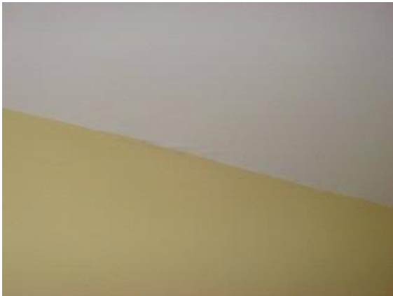
Bathroom #2 - 2nd Floor - Guest: View showing failing drywall tape
