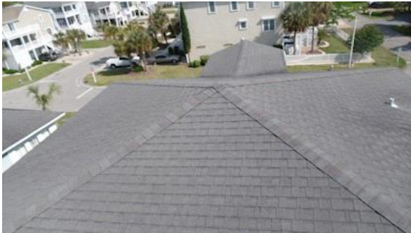
Roofing: Overall views of asphalt roof shingles
