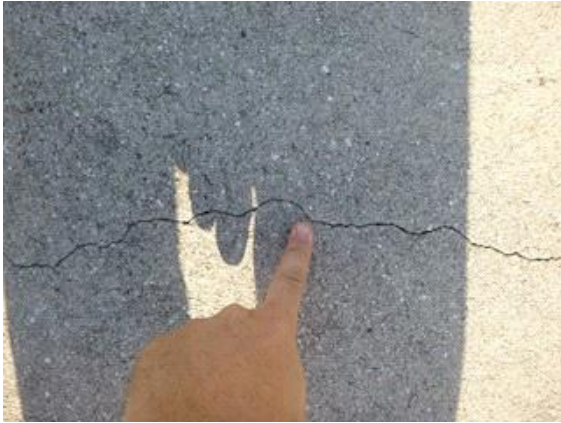
Driveway: View of minor cracks located in concrete driveway
