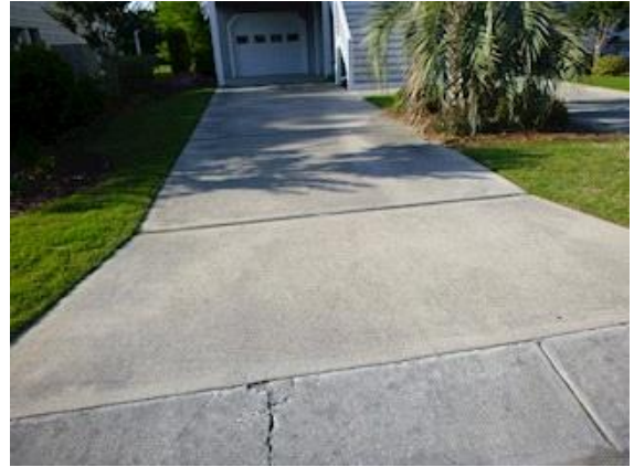
Driveway: Overall view of concrete driveway
