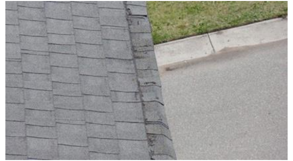
Roofing: Views showing missing shingles
