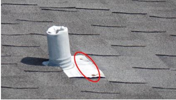
Flashing/Valleys: View of exposed nail heads at the base of vent pipe flashing
