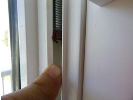
Living Room/Dining Area: View showing broken sash springs
