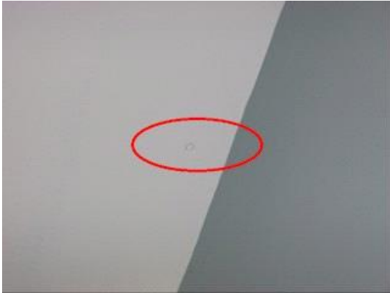
Bathroom #1 - 1st Floor: View of nail pop located on the bathroom ceiling
