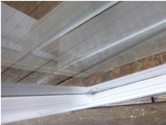
Exterior Doors: View showing rust between glass panes
