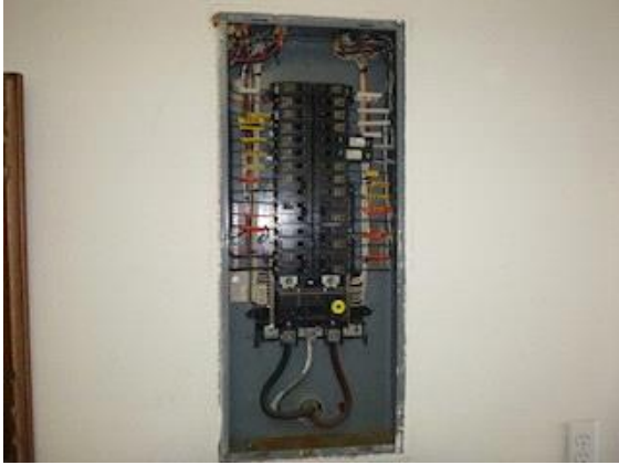
Electrical: View of main electric panel and circuit breaker located in the garage
