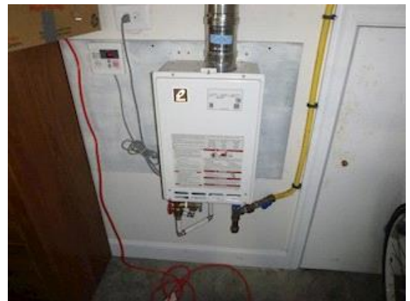
Water Heater: View of tankless water heater located in the garage
