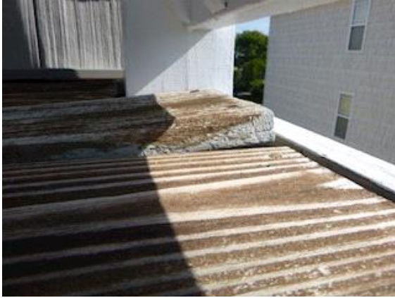
Decks - Rear: View of lifted deck board on rear wood deck
