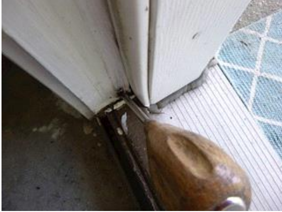
Exterior Doors: View showing water-damaged door jamb
