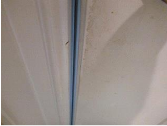
Garage Pedestrian Door into House: View of daylight shining through the garage pedestrian door
