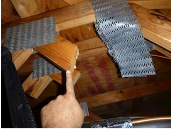
Attic Framing/Sheathing: Views showing cut roof trusses
