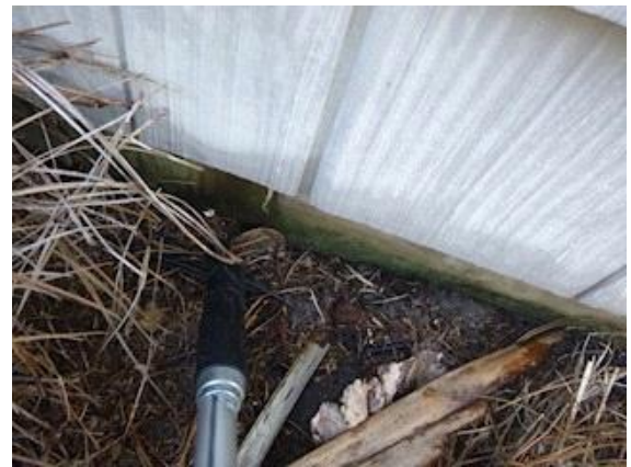
Under Floor Framing & Support: View probing the wood pilings at the base
