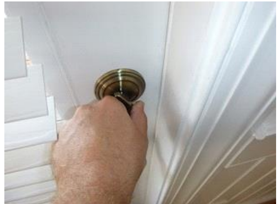
Exterior Doors: View of binding dead bolt
