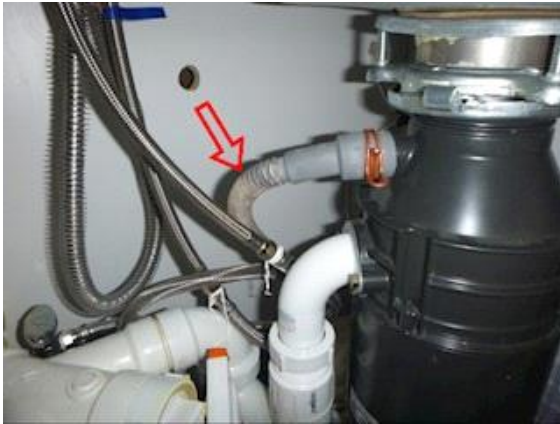
Kitchen: View of dishwasher drain hose with missing anti siphon loop located under the kitchen sink
