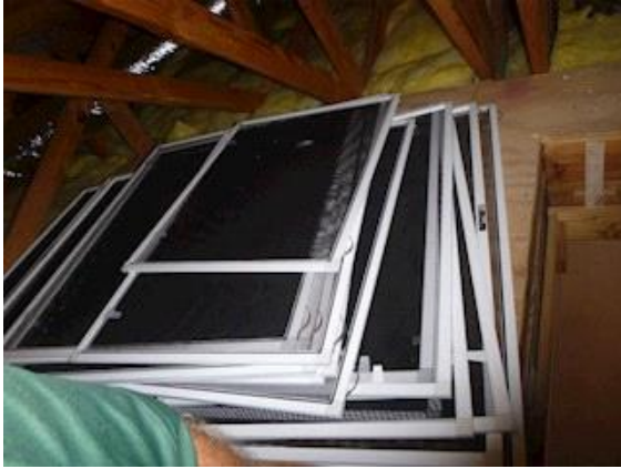
Windows: View showing the stack of window screens located in the attic area
