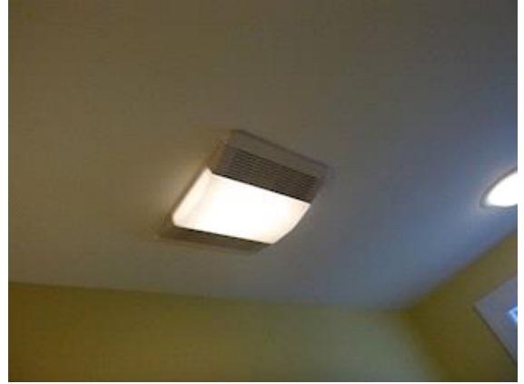
Bathroom #2 - 2nd Floor - Guest: View showing noisy exhaust fan
