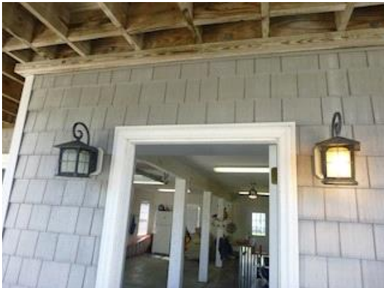
Exterior Surface: Views showing defective exterior lights
