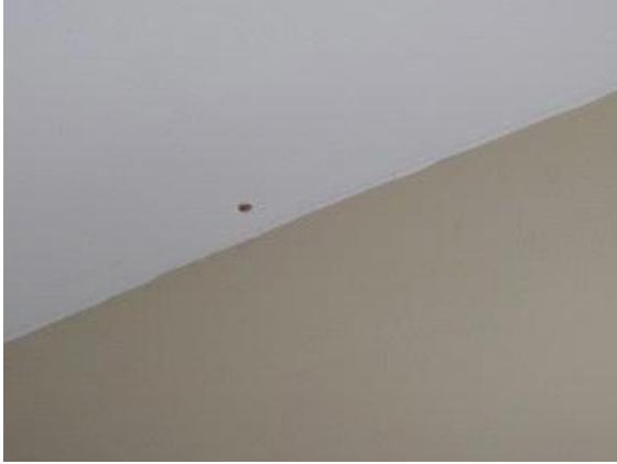
Bathroom #3 - 2nd Floor - Master: View of nail pops located on the bathroom ceiling
